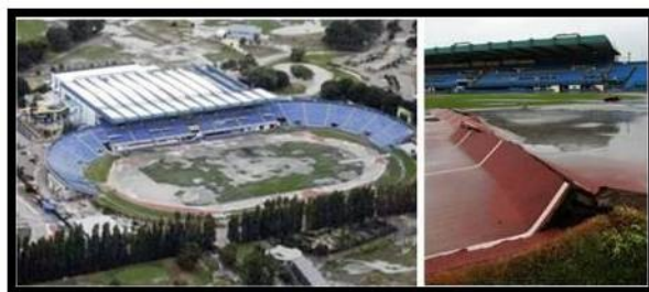
QEII stadium showing liquefaction (left) and damage to the athletics track (right) following the February earthquake.
